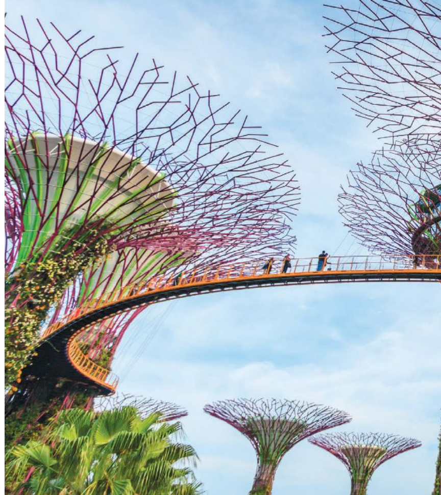
Supertrees at Singapore's Gardens by the Bay. The tree-like structures are fitted with environmental technologies that mimic the ecological function of trees.
