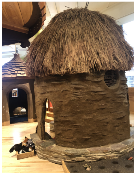
Fig. 3. These Wildernest play huts are made from wheat straw, soil, linseed oil, and wood.
