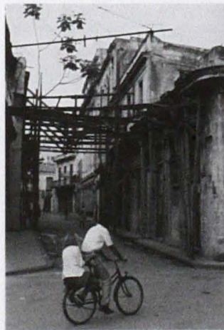
Wooden beams help keep buildings from falling on Plaza Vieja in Havana. Photograph by Myriam Springuel.
